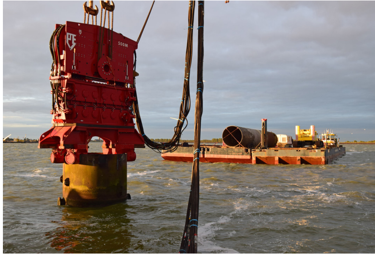
Figure 2.8: Vibro-driving system [46]
