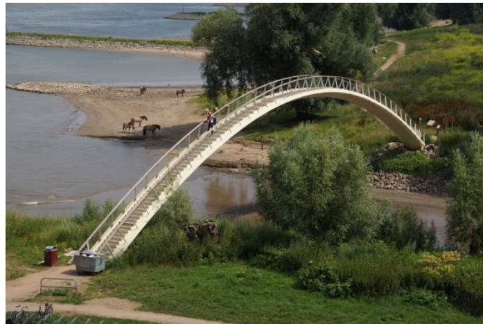
FIGURE 2.18 – Passerelle de Ooypoort
