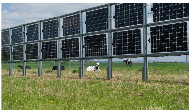
FIGURE I.9 – Structure fixe en acier. ©Next2Sun
