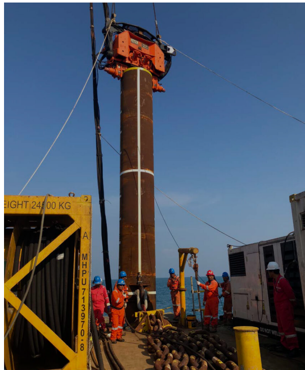
Figure 11: Example of offshore monopile installation by vibratory driving. Source: CAPE Holland [8].
