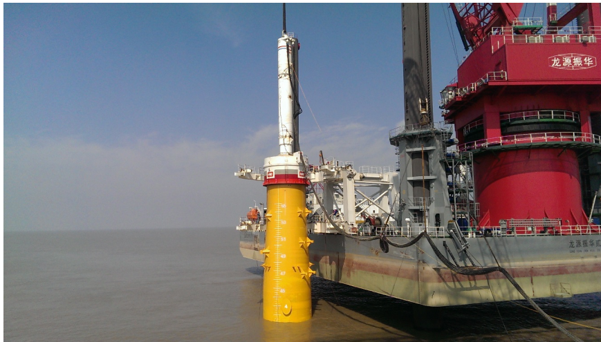
Figure 10: Example of offshore monopile installation by impact driving using a hydraulic hammer. Source: Offshore Wind Biz [7].
