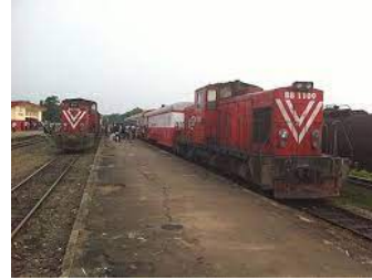
(b) CAMRAIL Railway Network outdated infrastructure [27].
