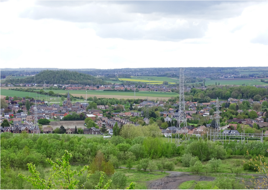
Fig. 25 - View from the power station from the Quesnoy slag heap, 2024
