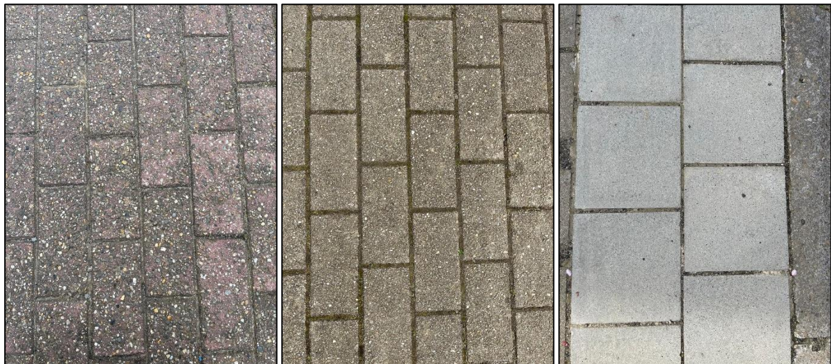
Figure 29 : Different types of concrete pavement captured in Louvain-la-Neuve
