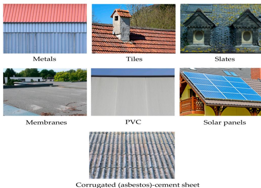
Figure 9 : Example of the 7 different classes of roof type from the WaRM (Wyrd, 2023)
