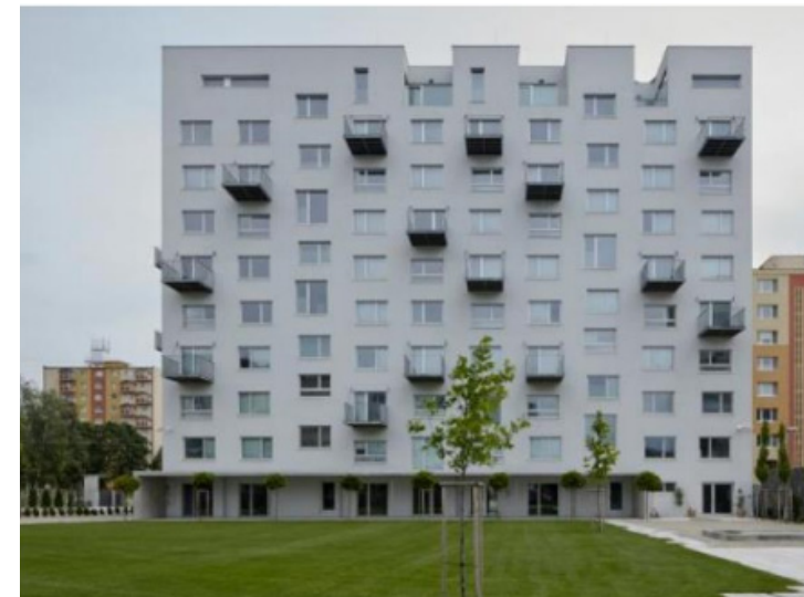
Fig 83. Building after the renovation work
