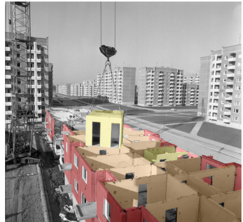
Fig 28. Assembly of the various elements into prefabricated panels using cranes on rails. Source: initial photo made by Bernardas Aleknavicius 1987-1988.
