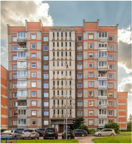
Buildings with 10 floors
