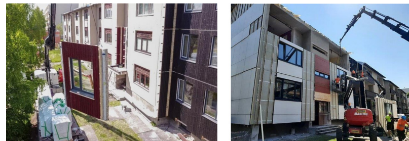
Fig 118. Renovation of an apartment building with new prefabricated panels, Estonia 2025. © Svetaine.lt Assembly of the prefabricated panels, 2024. © Lrt.lt
