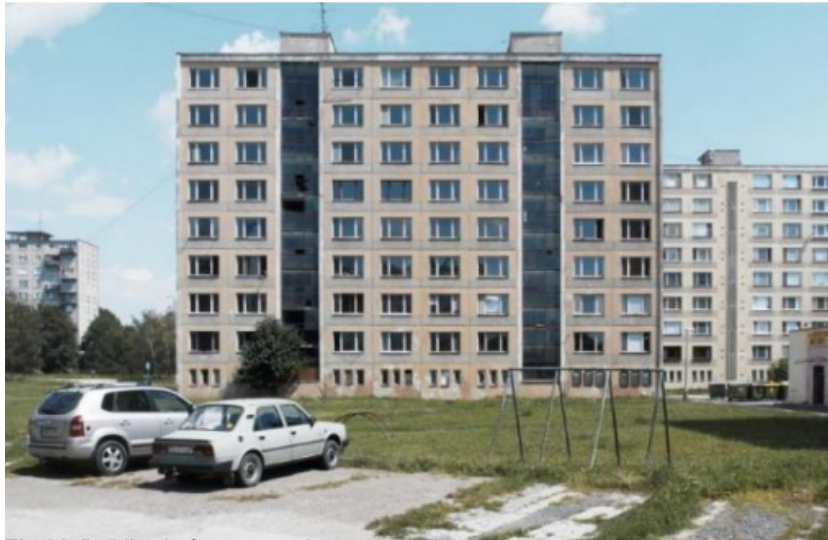
Fig 81. Building before renovation work
