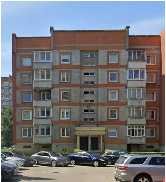
Buildings with 5 floors
