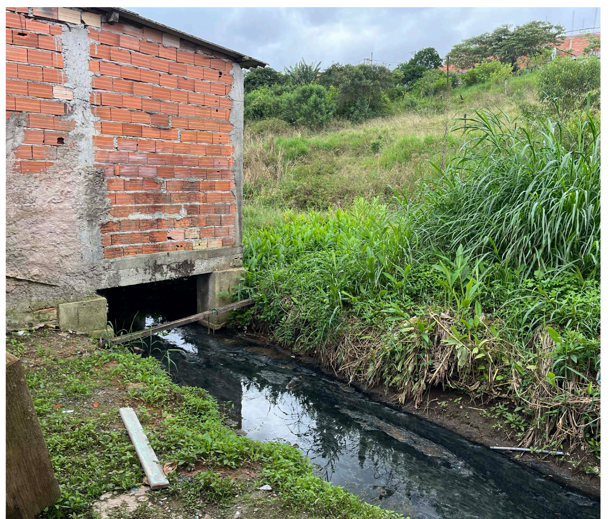
Sewers running under dwellings
