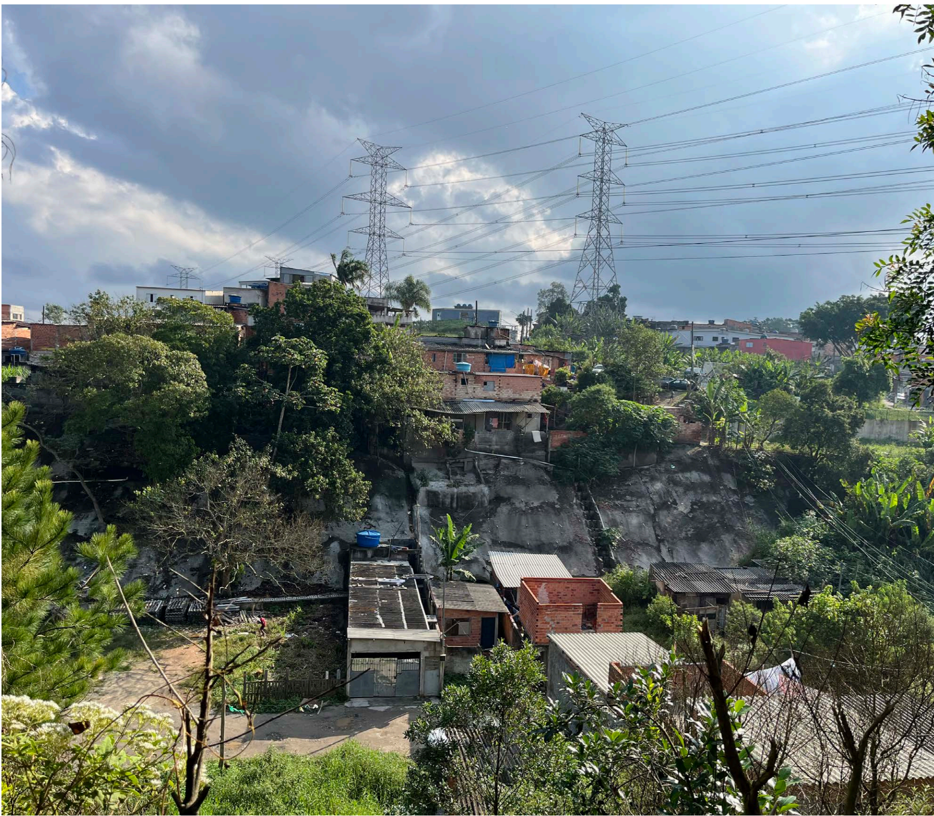
Government-built drainage system
