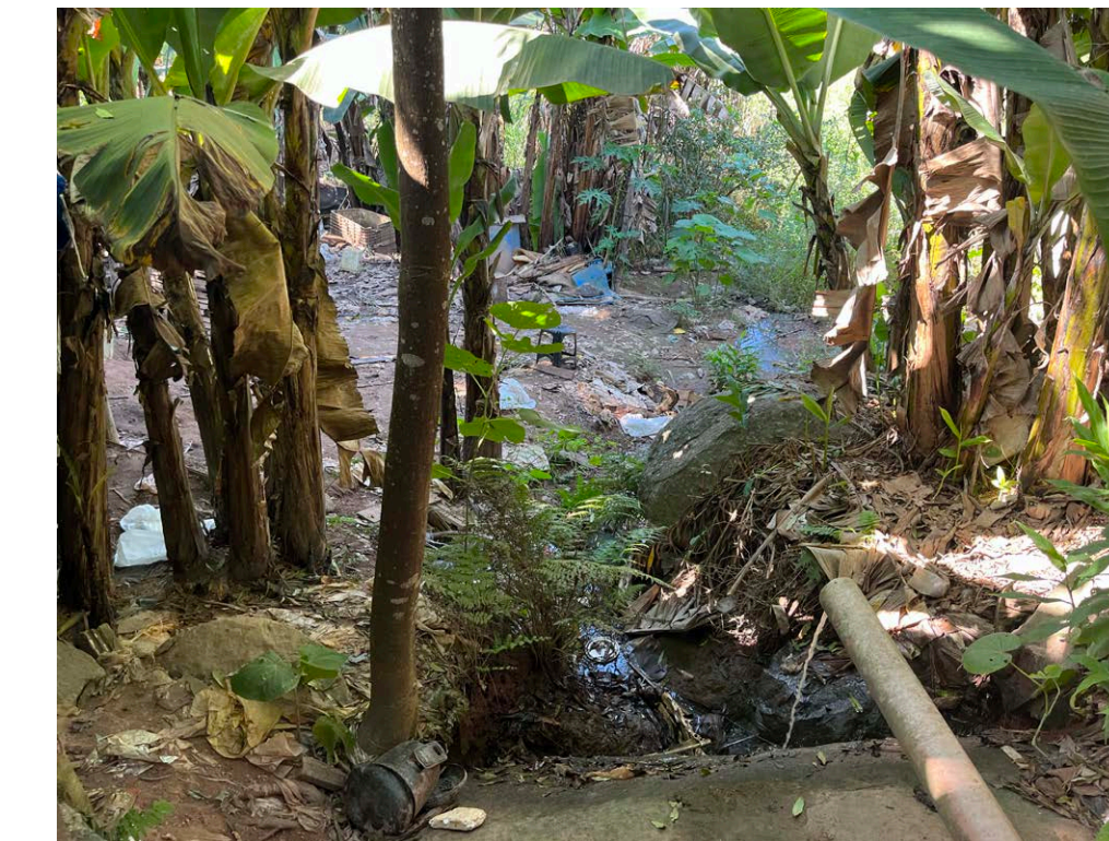
Runoff drain pipe discharging into the lake
