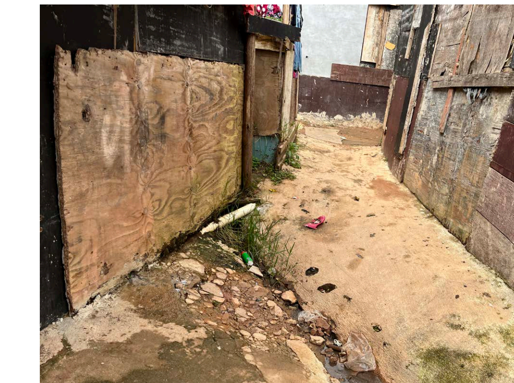
Runoff flowing beneath Ilana's house
