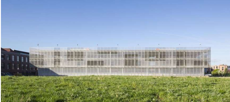
Fig.17 Parking-silo mutable de la Plaine Image
