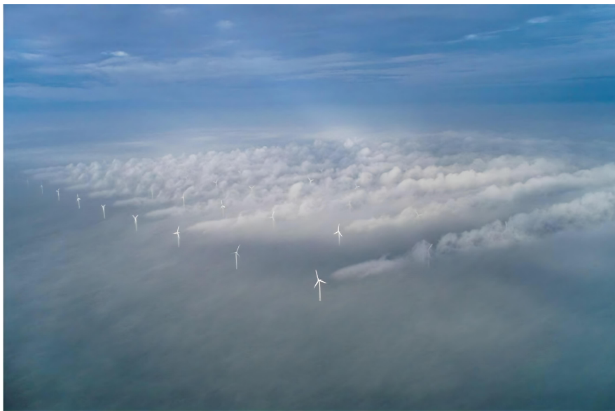
Figure 1.1: Horns Rev 1 offshore wind farm property of Vattenfall - Photographer Christian Steiness.
