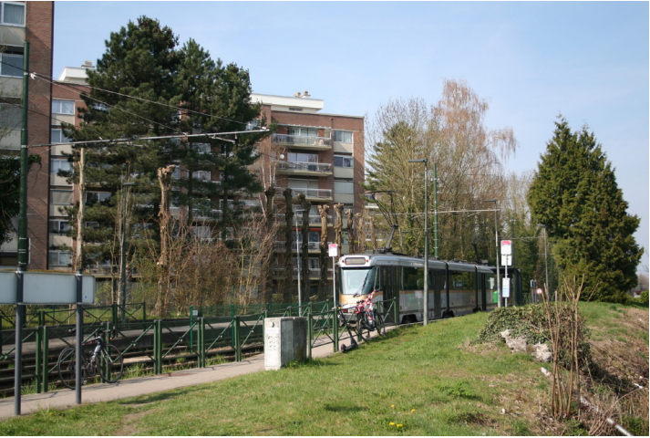
Station Ban-eik à Wezembeek Oppem. Figure 70
