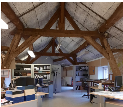
Annexe 28: Combles (bureaux)
