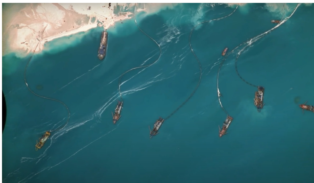
Chinese ships taking sand from the sea ground and moving it towards the reefs to elevate it above the sea level
