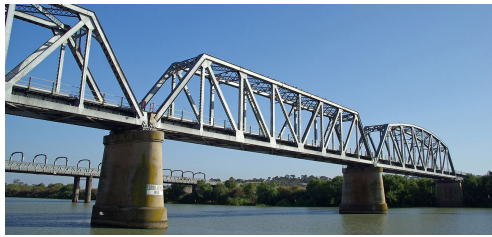
(a) Photograph of a truss [32]
