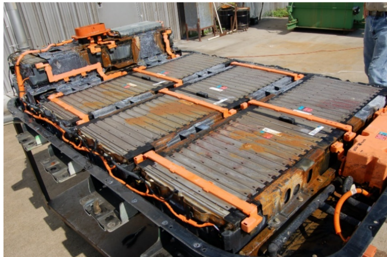
Figure 4.6: Degradation at the pack level
