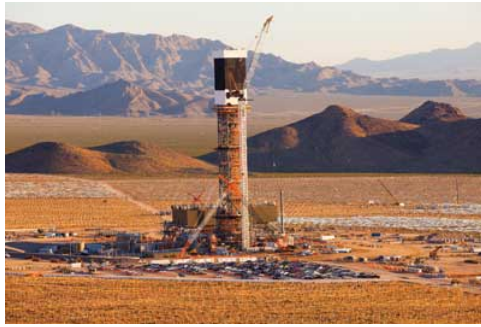
Example of bare area. Ivanpah CSP tower construction (USA), source http://www.powerengineeringint.com
