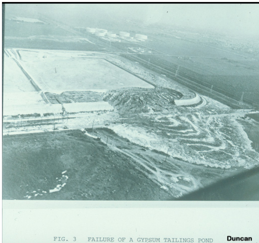
Figure A.2: Aerial view of such tailings dam failures. The picture comes from (Geotechnical Photo Album, University of California Davis 2025)
